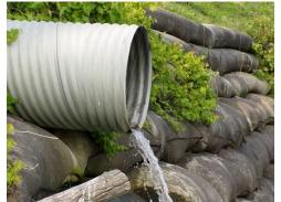
Systems designed to discharge may not exhibit obvious signs of failure. If they discharge to an underground collector pipe or storm sewer, the improperly treated sewage and resulting odors may not be noticeable to the homeowner.
